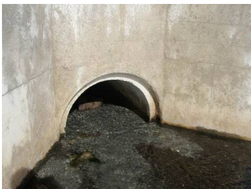
N4 – 10/2015 (exutoire pluvial)
