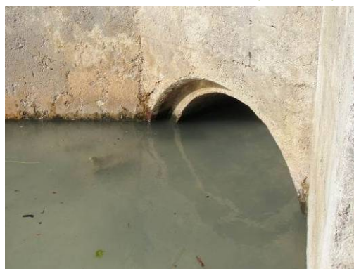
N5 – 10/2015 (exutoire pluvial)
